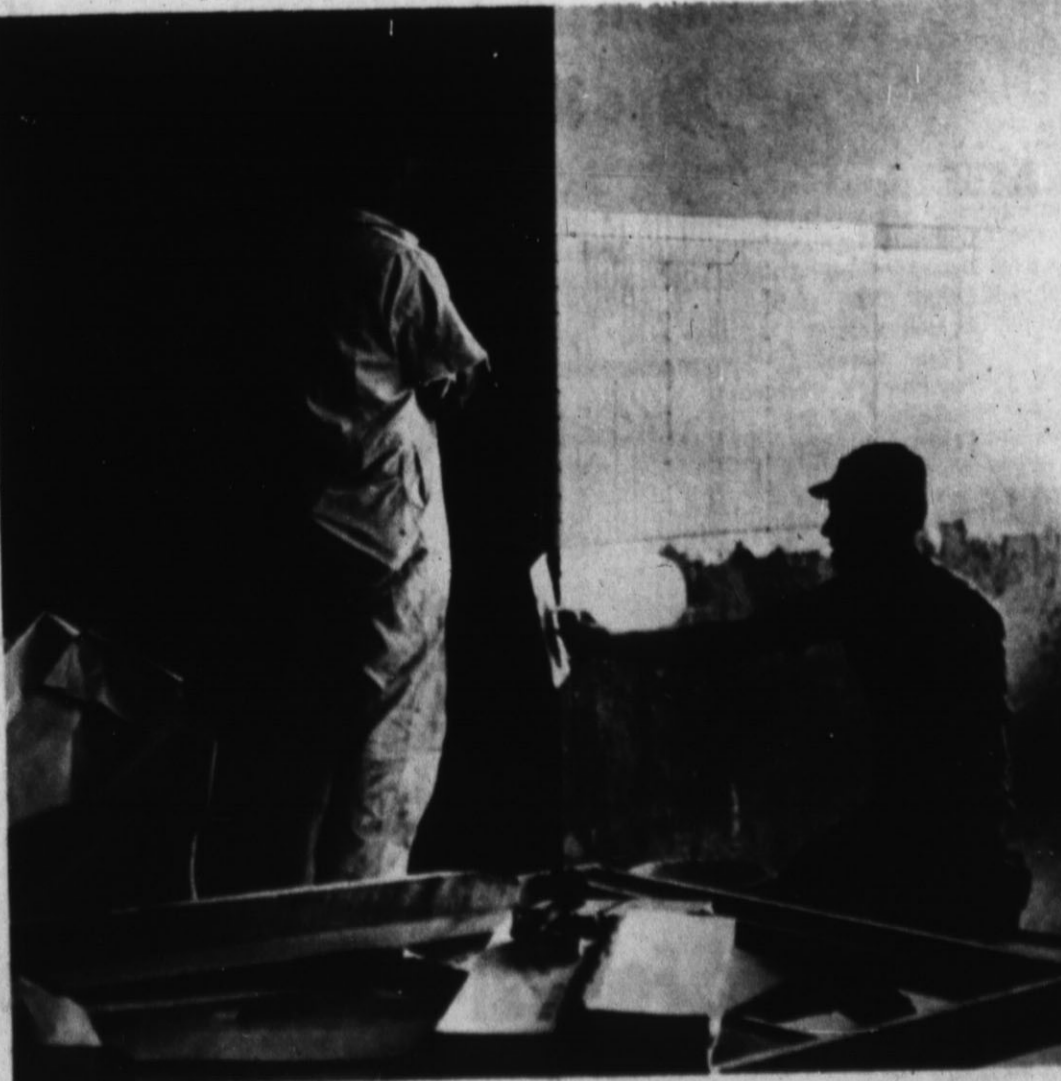
Workmen apply tile at Bluebonnet School.
