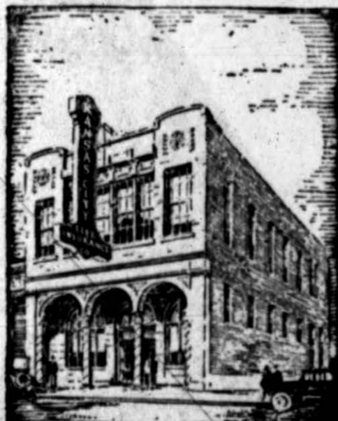
The O. Sam Cummings Agency Building, Dallas
