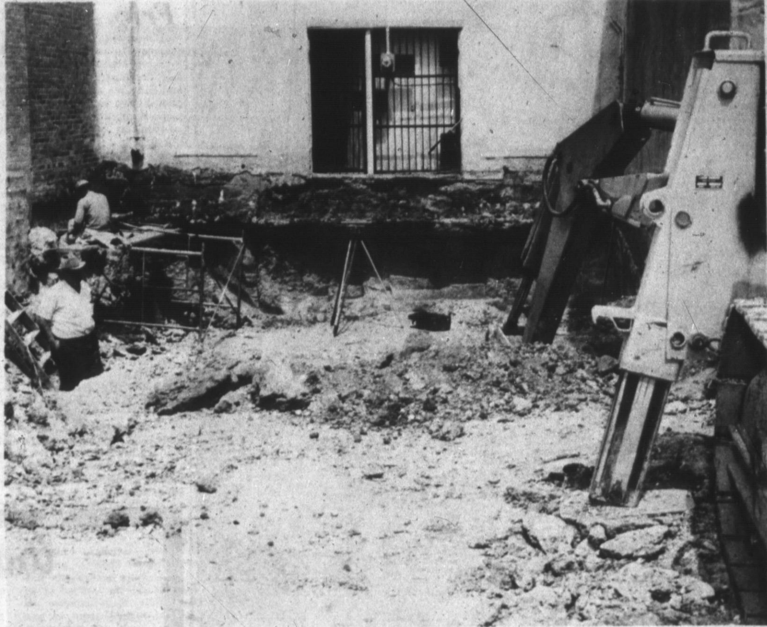
NEW BASEMENT — This is part of the construction which is taking place at the Popular Store on Main St. The store will be extended to the alley and there will be upper and lower levels to the new additions in the store. This excavation is being made to allow for the split-level addition. (Brand Staff Photo)
