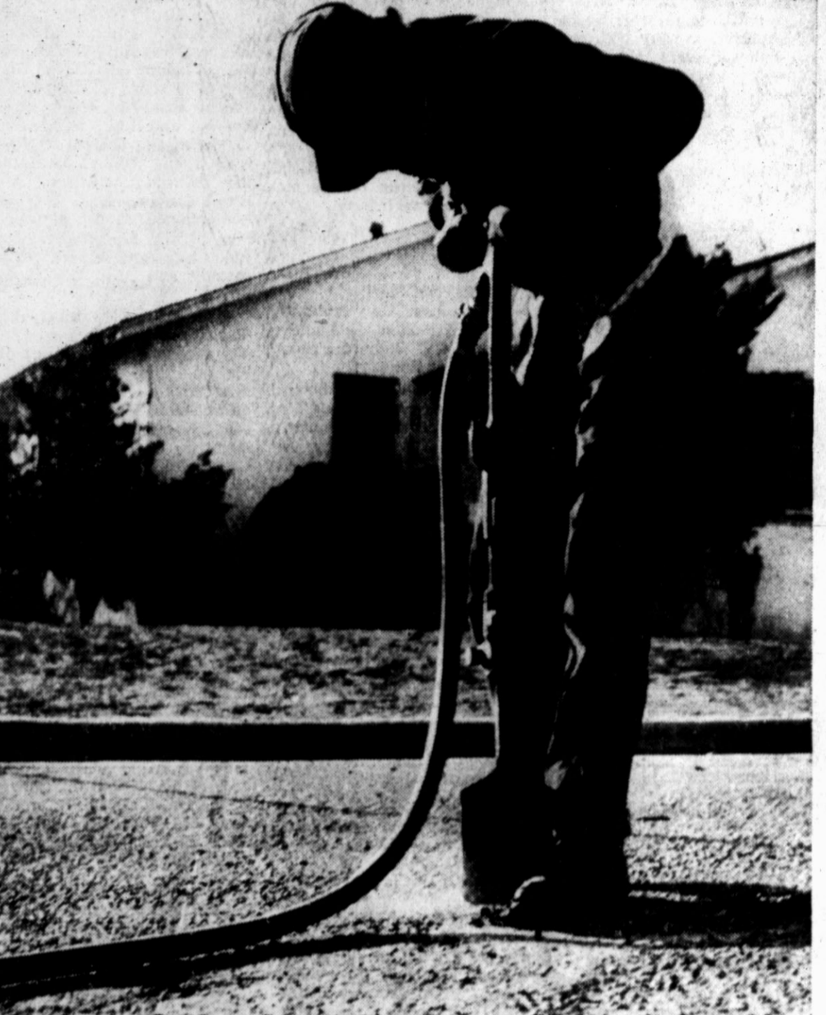
REPAIRING OF STREETS within Hereford city limits went into full swing this week after thawing of snow last weekend. Alternate freezing and thawing of ice this winter created a great deal of work for the city street repairing crews, work which will continue through spring and into summer. A city employee is shown operating a clay spade, powered by an air compressor unit purchased by the city recently. (Staff Photo)
