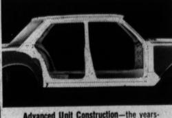
Advanced Unit Construction—the yearsahead breakthrough in car buildingwhere massive uniside members formed from one piece of galvanized steel (shown in white) replace scores of small parts
