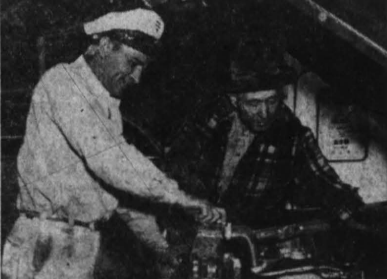
SOME SERVICE STATIONS need to be open all the time to take care of people who must have gas, oil or service. Odice Bulls and Tom Sanders were two of the men working at service stations in Hereford on Christmas. Both of them are at Pitman's, which doesn't even have a lock on the door. (Staff Photo)
