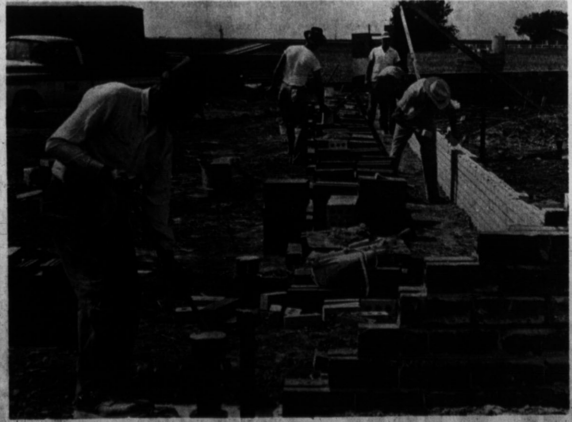
GENERAL OUTLINE of King's Manor retirement home in Hereford is beginning to be seen as brick walls go up. A spokesman for Knox and Gailey, Lubbock contractors who are building the structure, said that good weather had enabled them to go ahead of schedule. After a stone "bell" is laid, bricks will be used to complete the exterior walls. (Staff Photo)
