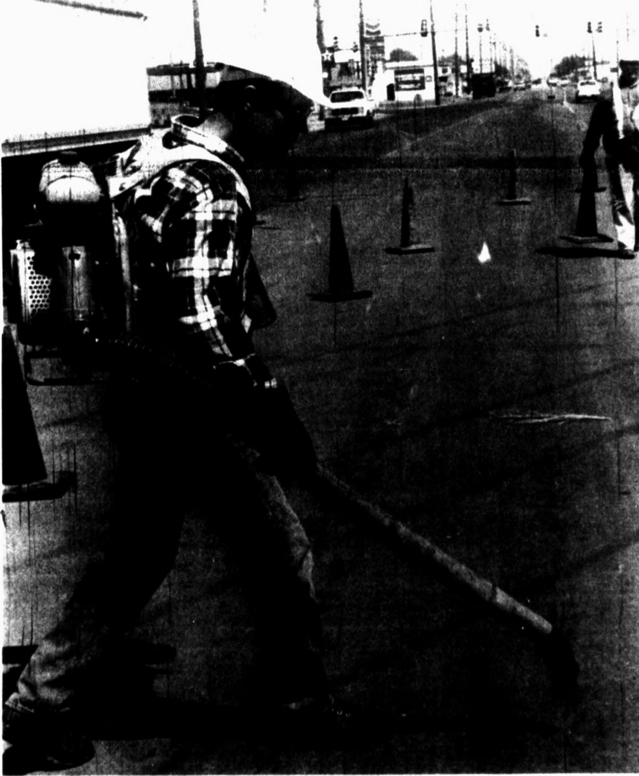
Ron Matthews of the Hereford office of the State Department of Highways and Public Transportation uses a back-pack compressor to clean dirt from cracks on West U.S. Highway 60 in Hereford. Road crews sealed cracks in the roadway on Wednesday.
