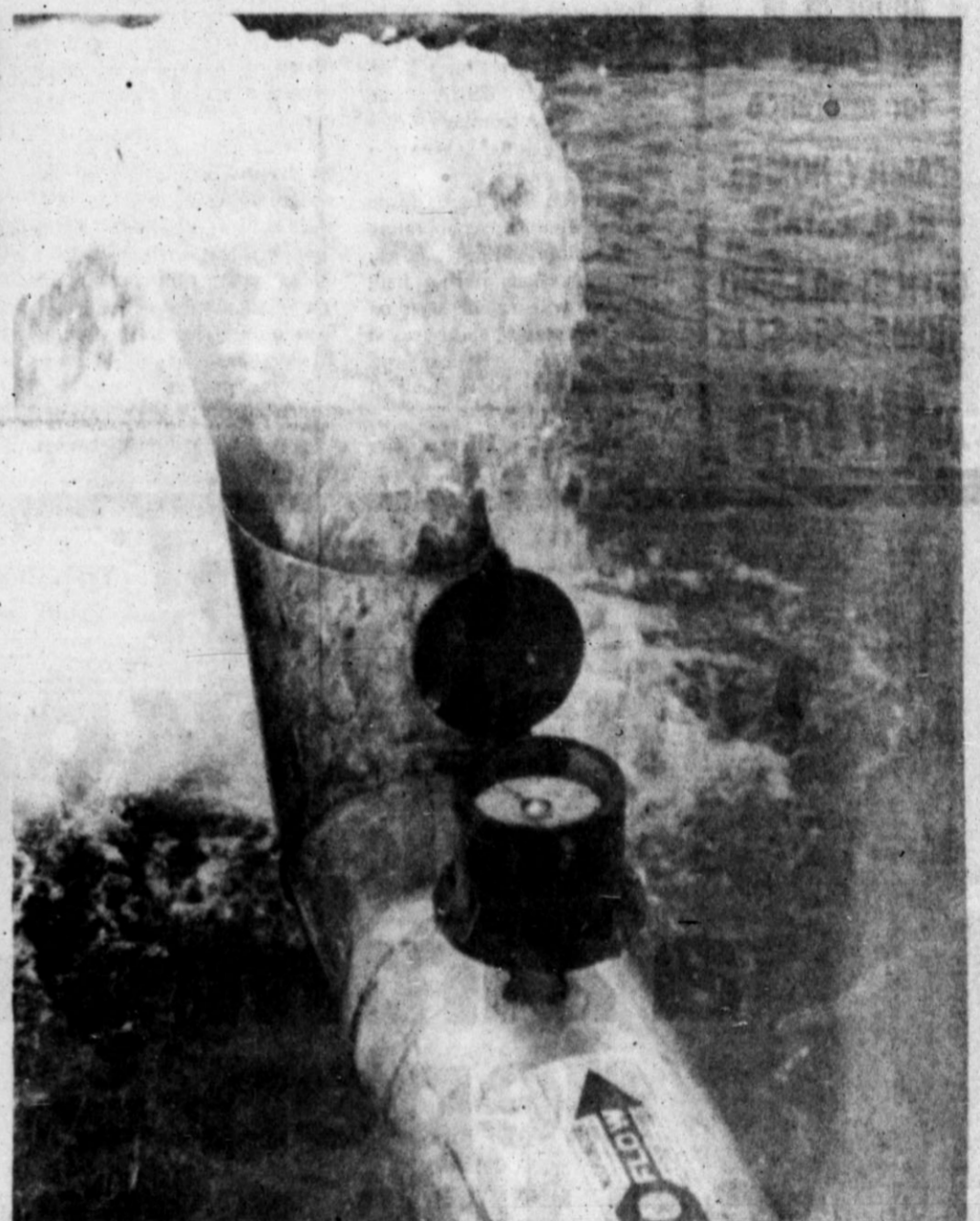
The discharge pipe and water meter tell the amazing story of a carefully-developed well. A pumping unit which delivers 1,100 gallons of water per minute—sand free. The use of a special drilling compound and uniform gravel trucked in from Colorado were two of the key factors in eliminating a sand pumping problem. Although costs for developing such wells are higher than normal wells, extra productivity with reduced pump wear should more than offset these factors.
