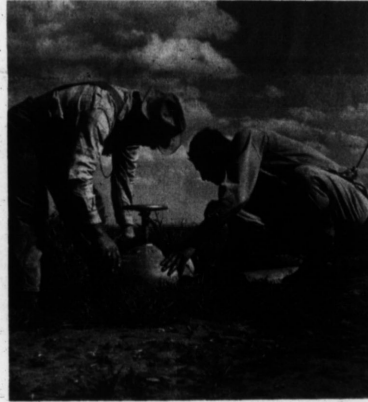
UNDERGROUND PIPELINES not only add convenience to farming, but are considered a valuable aid in water conservation. Frank Bezner and Tino Cortez set a value on one of the Bezner wells southeast of town.
