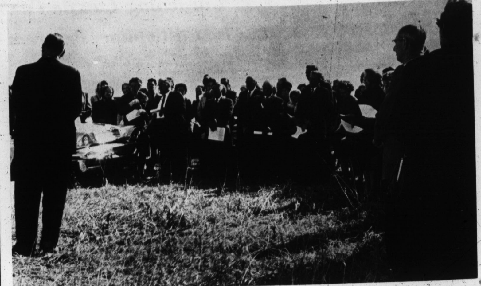
A LARGE CROWD GATHERED, despite windy conditions, when the official groundbreaking for King's Manor, a home for older adults, was conducted at the building site Friday. Along with many from Hereford, the crowd included delegates from many parts of the Northwest Texas Methodist Conference, which will administer the home.
