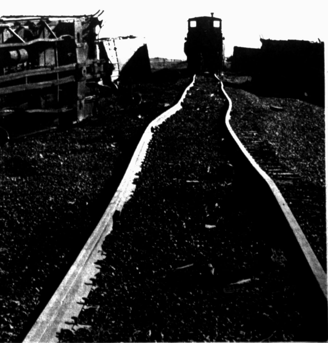
TWISTED RAILS show the force exerted when 11 cars of 132-car freight derailed Sunday morning. Tumbling to both sides, the cars left a quarter mile of track looking as if it had been twisted. No one was injured in the accident. (Staff Photo by H. A. Tuck)
