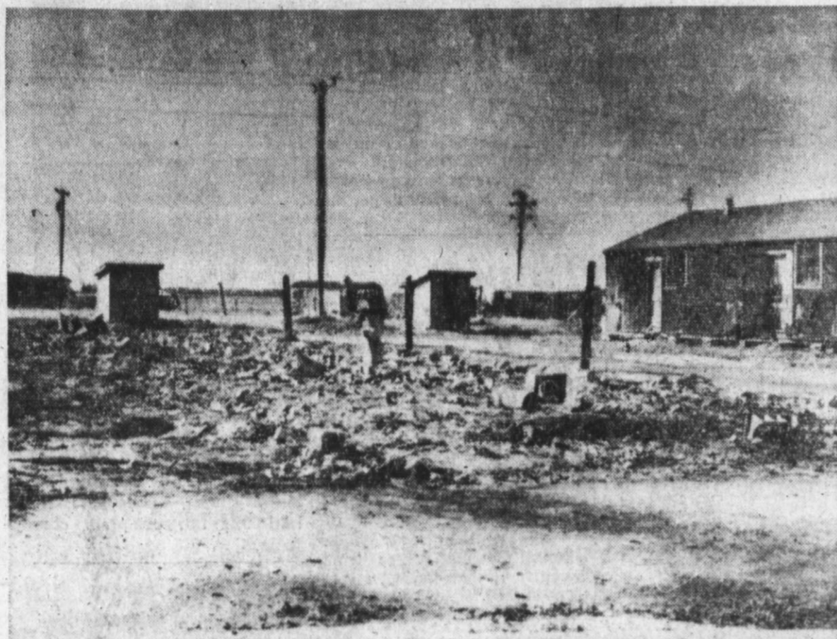
ASHES AND FOUNDATION blocks were all a small boy (center) found Wednesday as he wandered through what remained of an empty barracks building at the Labor Camp. The structure was struck by lightning Tuesday night and quickly was reduced to rubble as firemen concentrated on preventing the fire from spreading. (Staff Photo)
