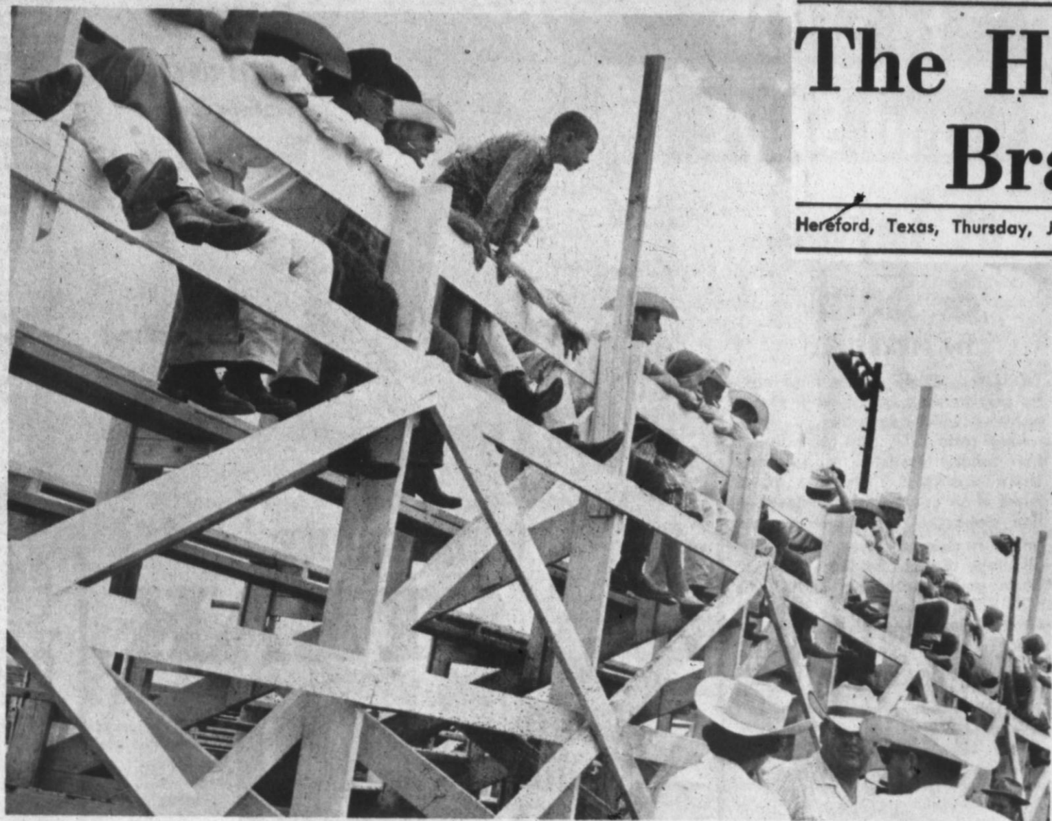
Boots were much in evidence among spectators
