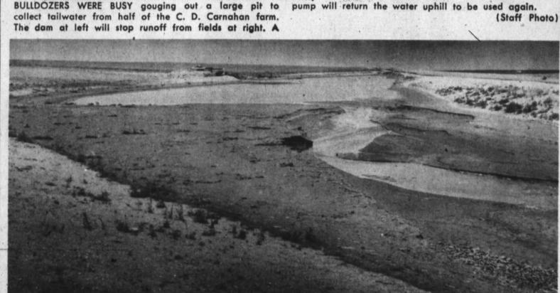
COMPLETED POND NOW SAVES half the tailwater on flows in from a series of ditches and channels. the Carnahan farm. The dock - mounted pump at the right of the reservoir works continuously on the tailwater that
