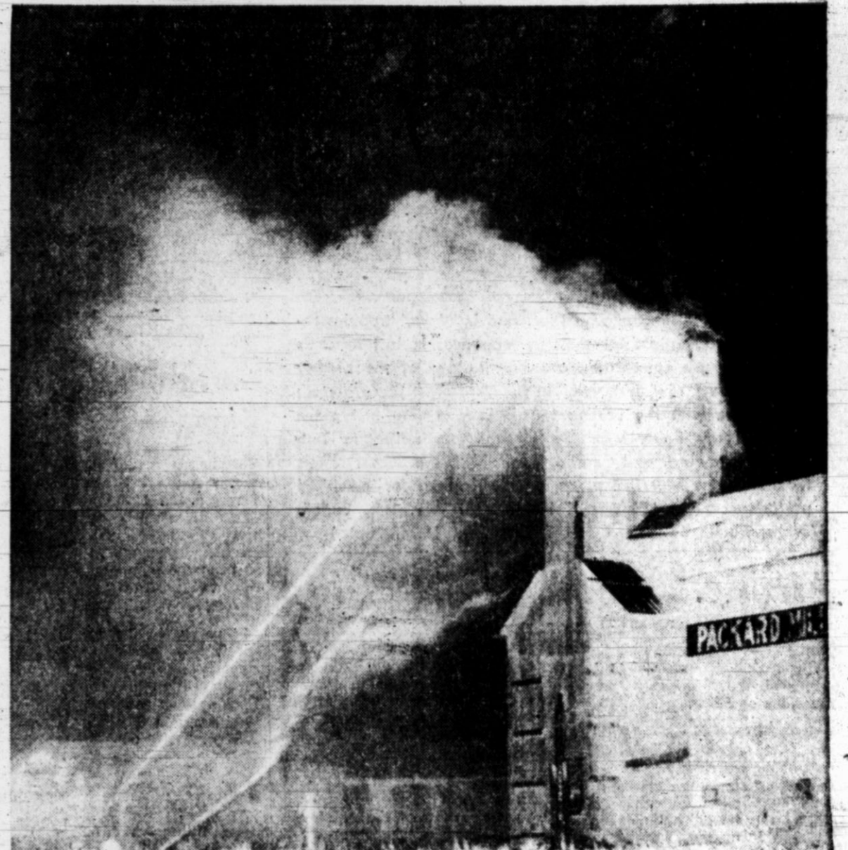
GRAIN ELEVATOR AFLAME —Fire had raced through the roof of the headhouse 60 feet above the ground at the Packard Milling Co. elevator Tuesday night before firemen arrived to bring their hoses to bear. Fire damage was confined to the high structure and its equipment. Only 4,000 to 5,000 bushels of wheat was in the structure, which was being cleared for the coming milo harvest. (Staff Photo)
