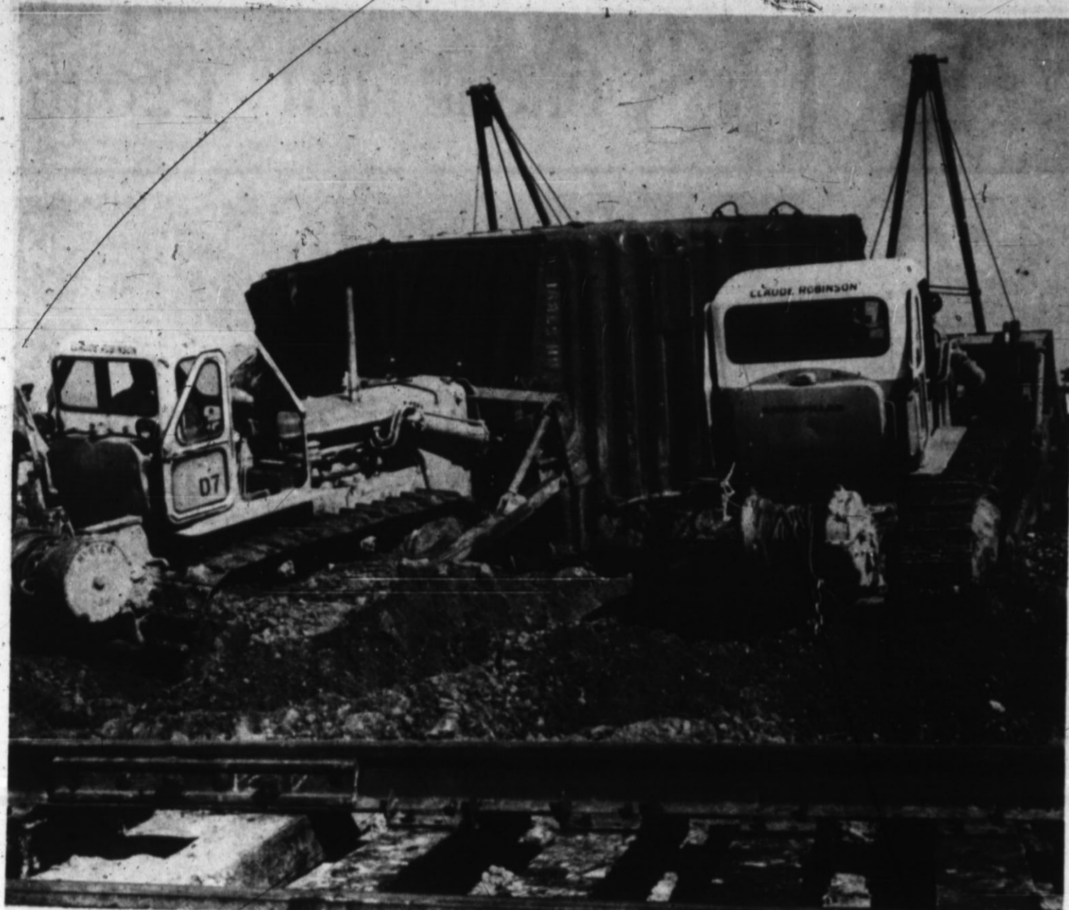
BULLDOZERS AND WINCH TRUCKS struggle to push and pull one of the 40 box cars which derailed seven miles southwest of Hereford on the main Santa Fe line to the West Coast. The wreck, which occurred about 12:30 a.m., was blamed by railroad officials on a faulty journal. As
