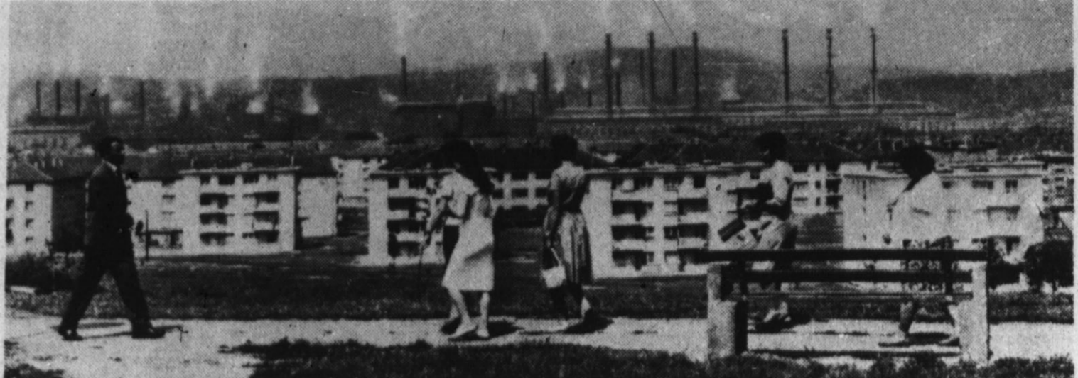
NEW APARTMENT HOUSES blossom in front of a steel plant at Hunedoara in Romanian Transylvania. This is typical of many new towns that have sprung up in Romania in recent years.
