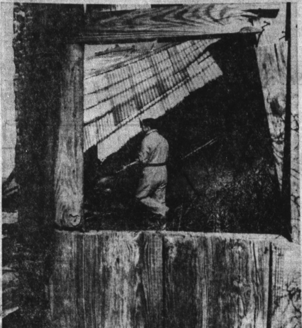
FRAMED by a charred barn window, Bill Howard, member of Hereford Volunteer Fire Department, helps extinguish a fire which destroyed a barn 2 1/2 miles northwest of Hereford Friday morning. The barn was located on an unoccupied farm owned by T. L. Kimball, 507 Ave. K. The blaze apparently started from a grass fire of unknown origin. No estimate of damage has been made. Firemen answered the alarm at 11 a.m. Friday. (Staff Photo by H. A. Tuck)
