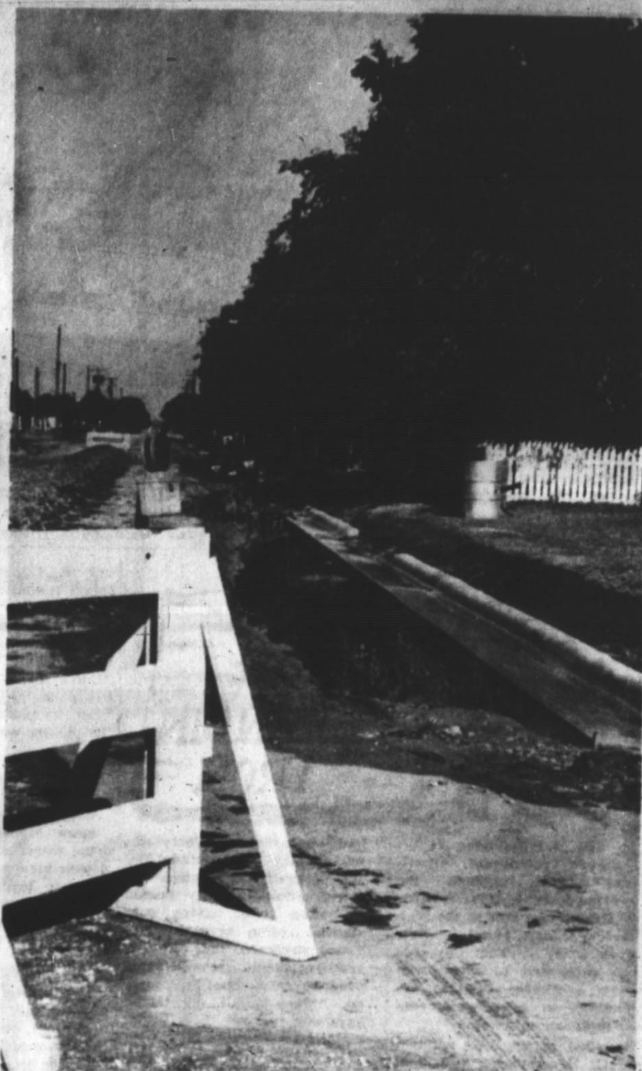
Construction work was slowed by the downpour.
