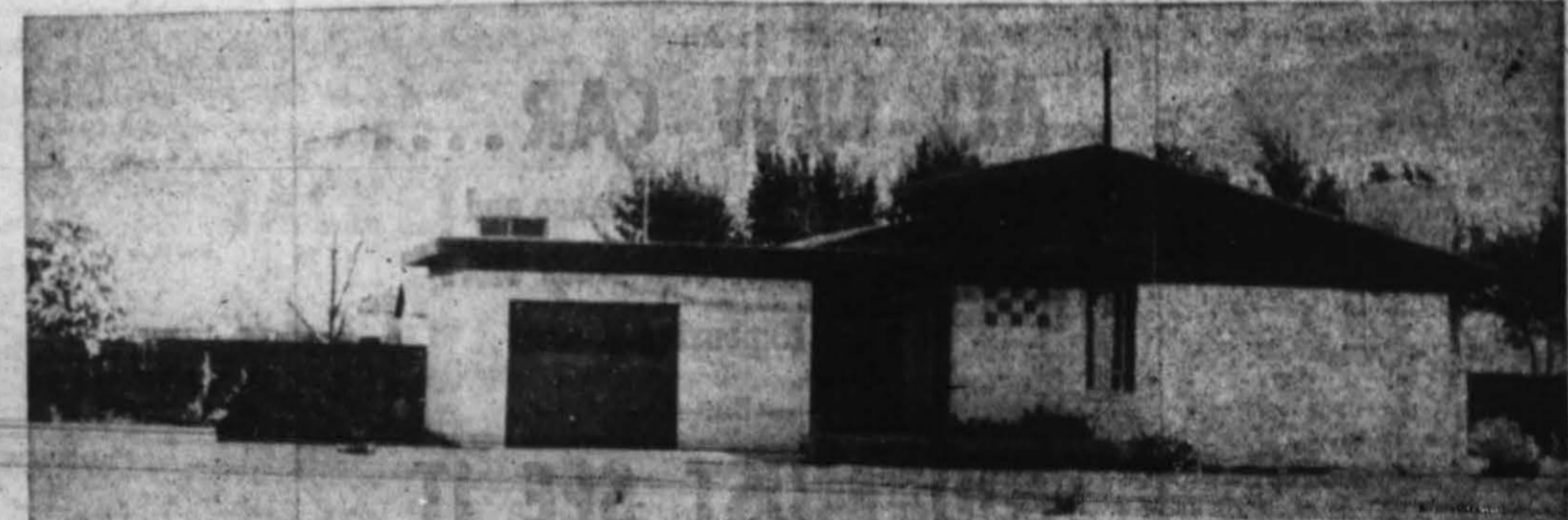
TYPICALLY MODERN in design, the Ray Godwin home, 102 Beach Street, features Early American architecture inside with ceiling rafters exposed in the living and dining area. Walls of cinder blocks and redwood feature shades of green, Furnitu-
