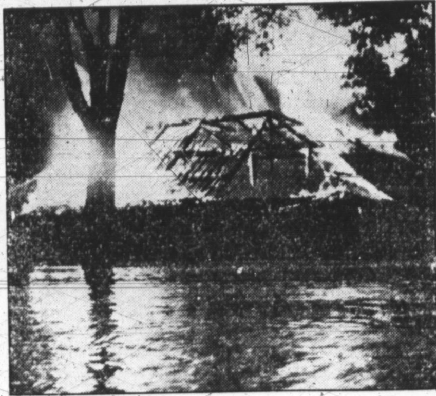
At height of the flood in Saffins, Kans., when the Spooky Hill river flowed three feet deep through parts of the city, fire broke out in Clafin Hall, city park recreation building, burning it to the level of the water.
