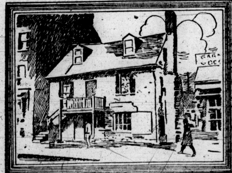
Washington's Headquarters While Directing Survey of Washington City, 1791.
