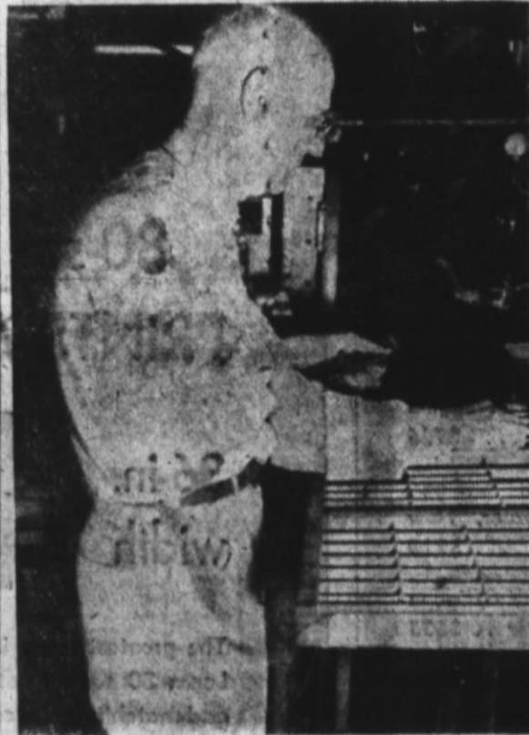
TAPE RUNS through the Linotype machine causing the letters to operate as if they were punched manually. Actual operation is highly similar to an old-fashioned player piano.
