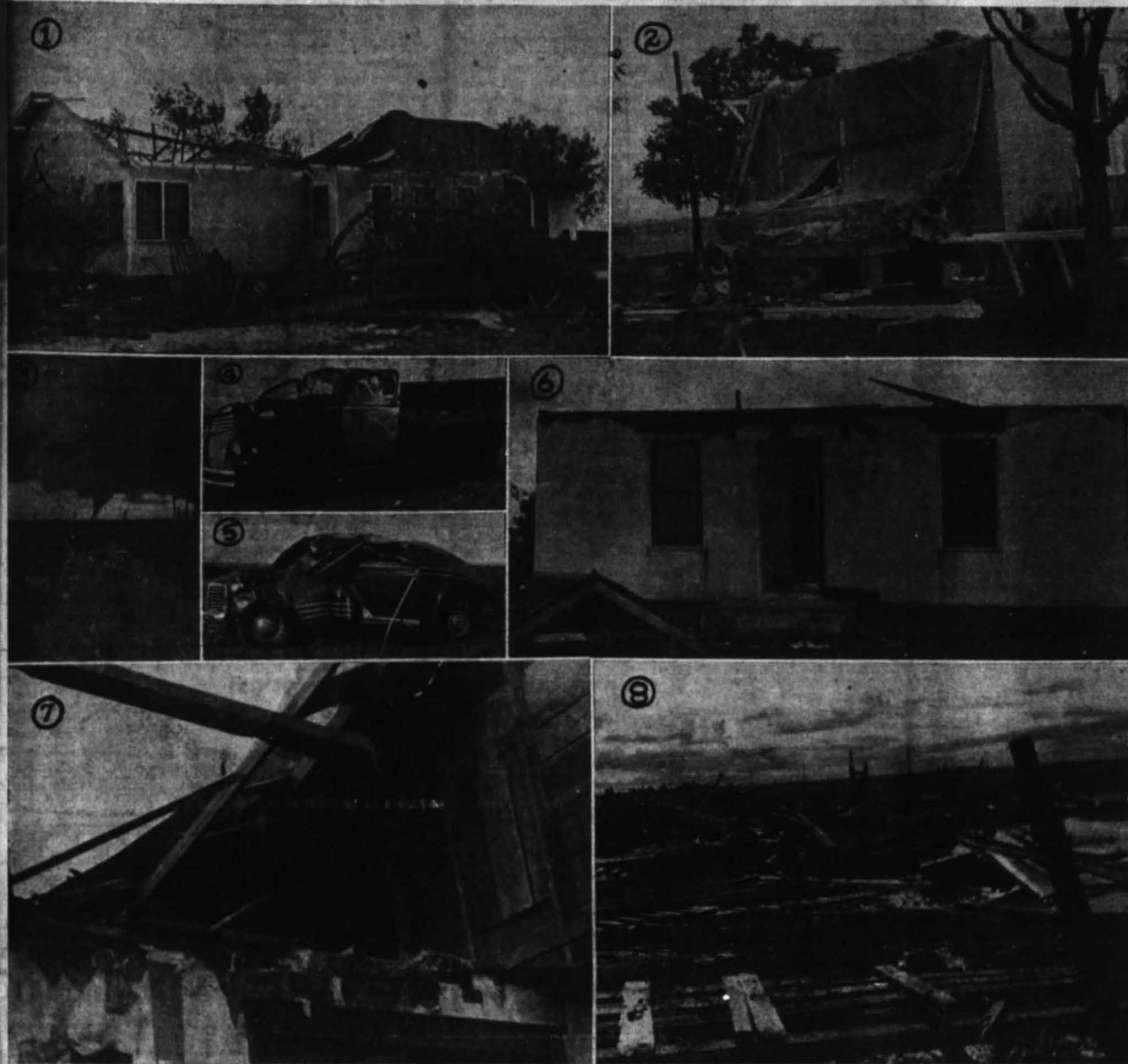
PICTURED ABOVE ARE SCENES OF DESTRUCTION in the path of the tornado which swept down Frio draw last week. (1) The Lee Cocanougher house; (2) The Wirt Albracht home where repairs were already underway Thursday; (3) the twister, snapped in action from the T. J. Bradford farm at 5:30 p. m. Wednesday afternoon by D. Sanford; (4 and 5) Truck and car belonging to Lee Cocanougher, wrecked by the storm; (6) tenant house on the Cocanougher farm; (7) inside the Cocanougher house; and (8) wreckage of the Albracht barns and corrals. Photo-credits: Nos. 1-2-6-7-8 by Jap Dickerson jr.; No. 3 by D. Sanford; Nos. 4 and 5 by Ted Matthews.
