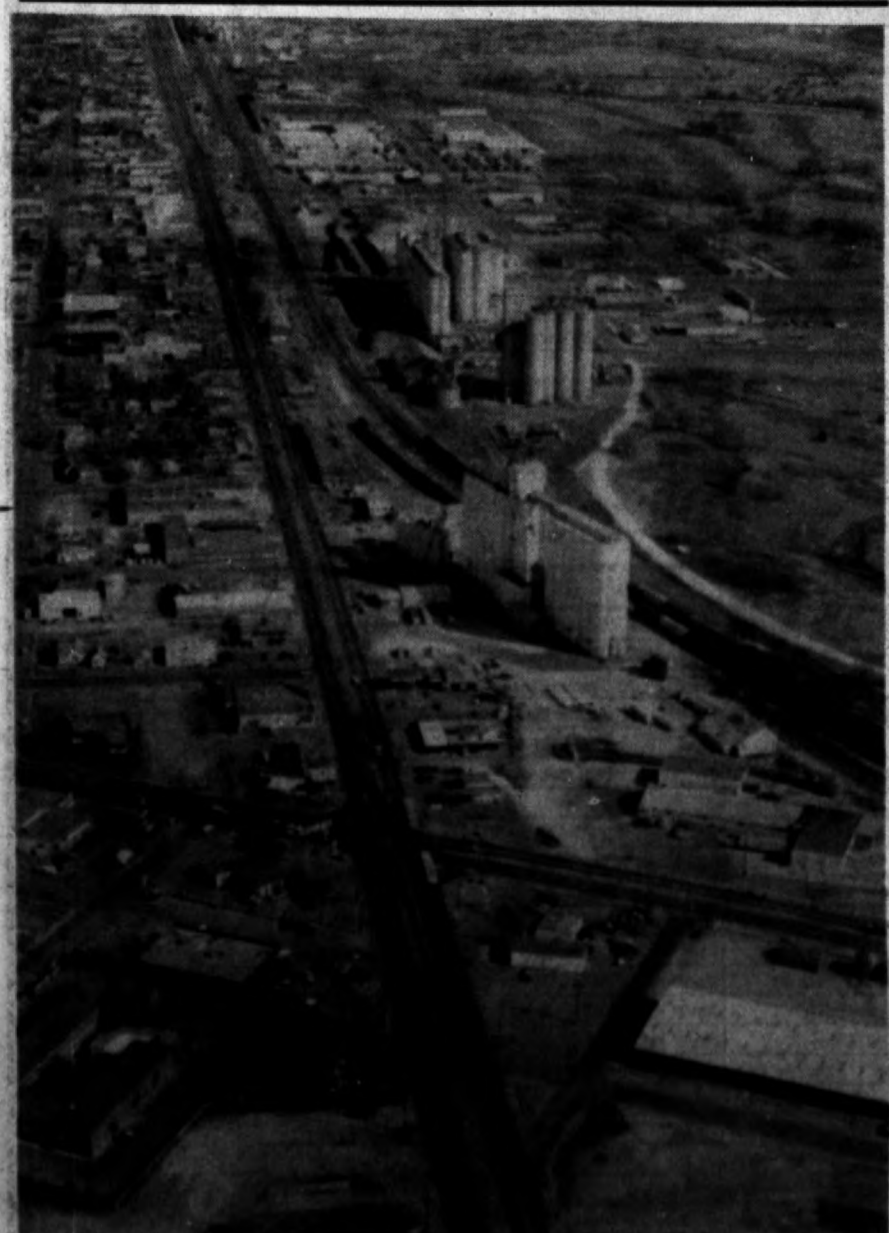
Aerial view of Hwy. 60 going through downtown
