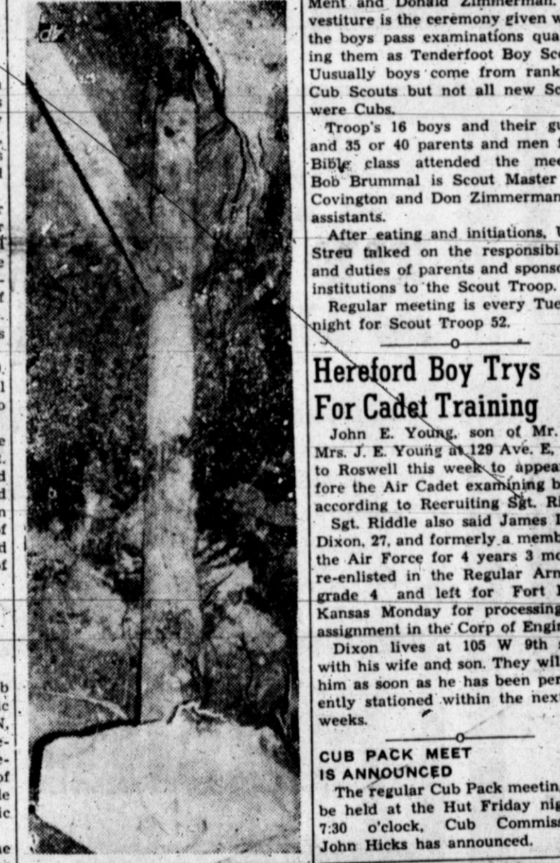
PIPE WHERE BOY WAS TRAPPED—Bobby Gow, 3, was trapped for 3 hours in the well casing shown above. After earth was dug from around the casing, workmen used cold chisels and heavy tin snippers to open the hole shown at bottom of well. The incident occurred at Austin, Texas. (AP Wirephoto)
