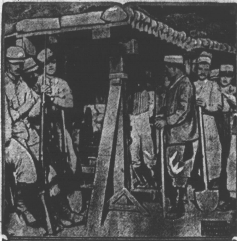
Men of the French engineer corps laying mines under cover of breast works at Belfort on the German frontier.
