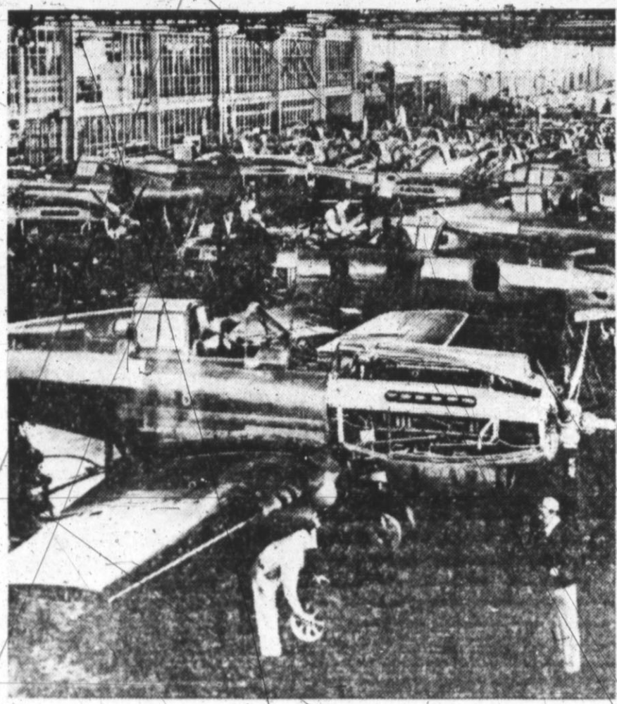
Mass production of the new Curtiss Tomahawk fighters for Great Britain's RAF new total a new high of eight planes per day at the huge Buffalo, N. Y., plant, a part of whose final assembly department is here shown. The Curtiss Tomahawk is the British name for the Curtiss Hawk 81-A "pursuit." The planes shown above will soon be England-bound.
