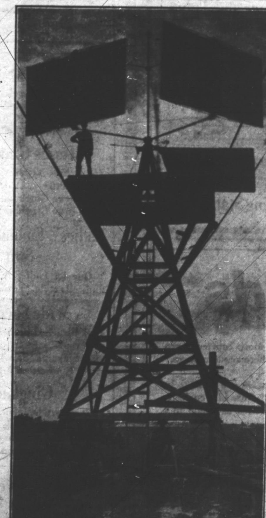
Robert Fullwood's Silent Automatic Windmill, which is now erected and in operation on the Schults farm in east Hereford. The power and promise of this new invention are causing widespread comment and favorable predictions from all who have examined it.
