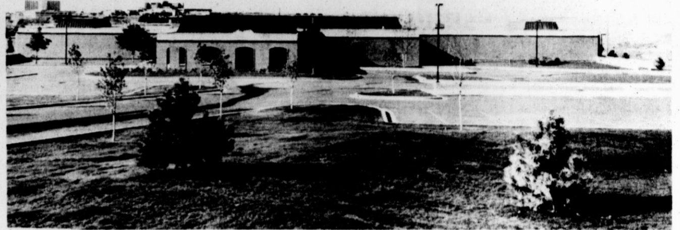
Clinic Expansion Completed
