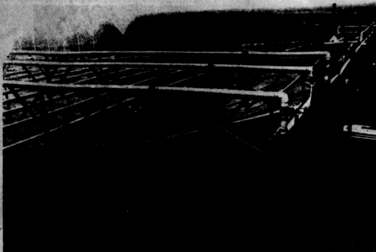
System uses winter cold to cool sprayed water and then stores it underground for summer use in air conditioning. Photo by John West
