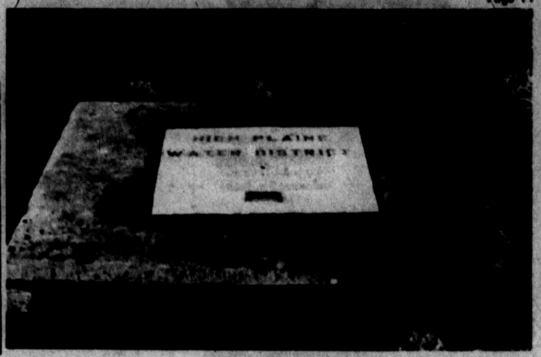
Plugged And Safe
