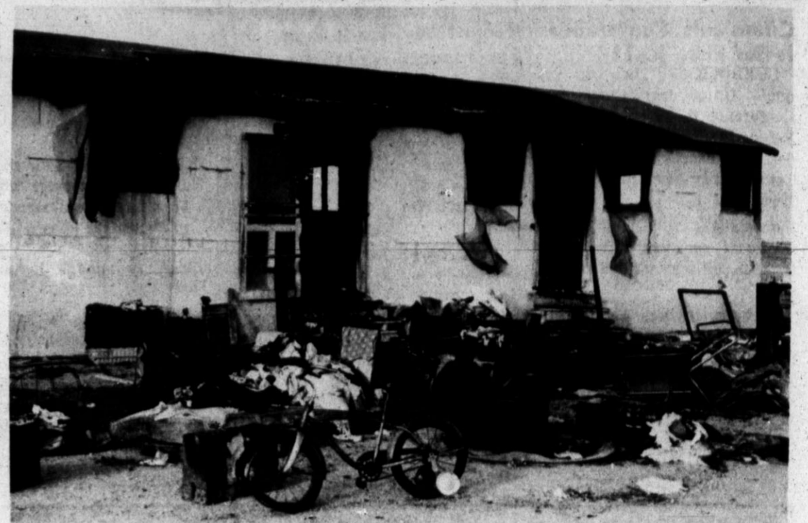
GUTTED BUILDING — Fire gutted this barrack building of Griffin-Brand one mile west of Hereford on U. S. 60 Sunday morning, causing damage estimated at $6,000. One person suffered injuries, described as minor, in the fire, which was believed to have started from a short in a light fixture.
