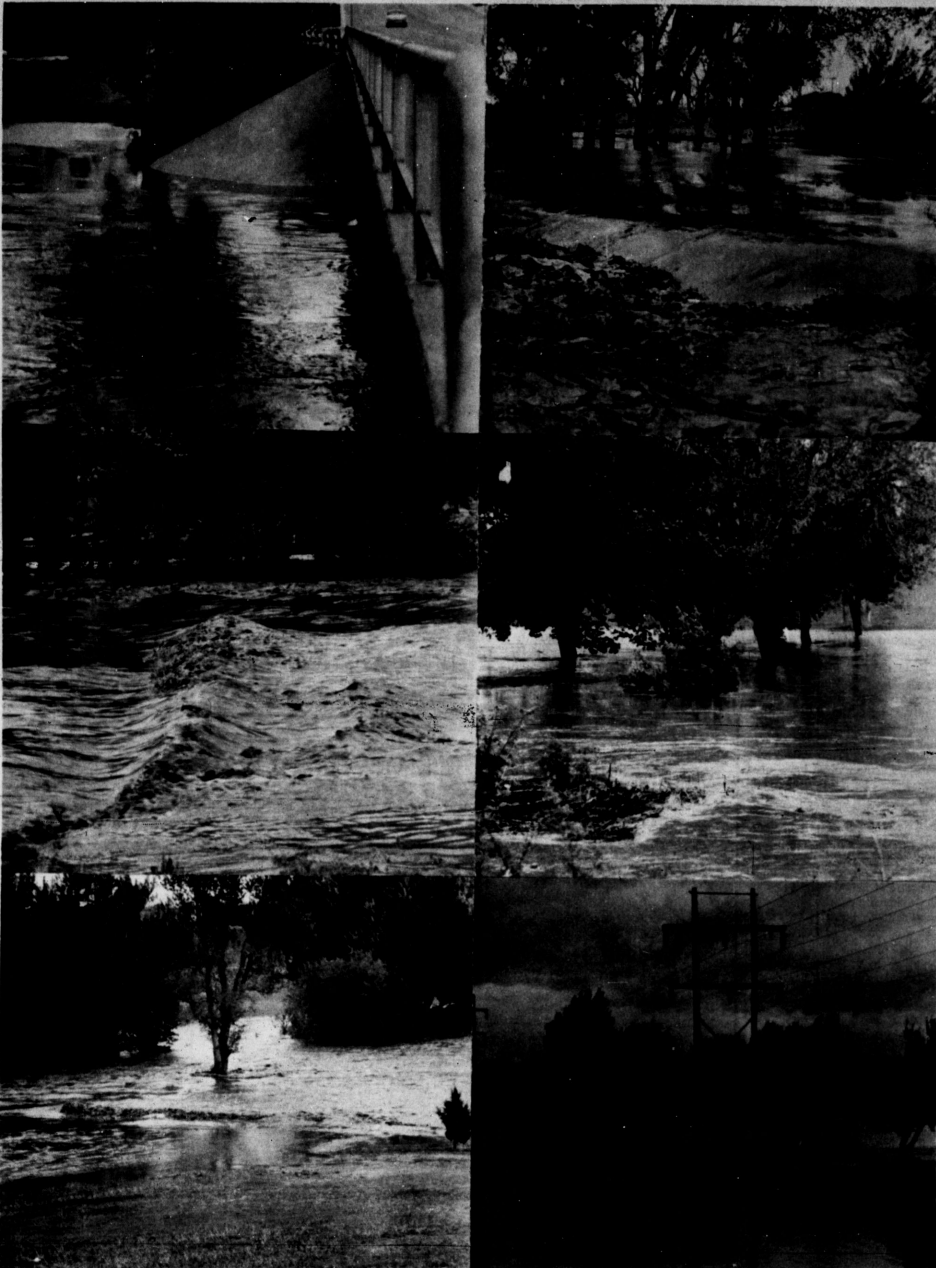
RAGING WATER — Rains throughout the week brought an abundance of water down the Tierra Blanca Creek from the watershed causing wide flood conditions at various points. In the top left photo, the bridge on South Main St. had a great amount of the water pass under it while in the photo in the top right, the Boy Scout Dam, located on the grounds of the Tierra Blanca
