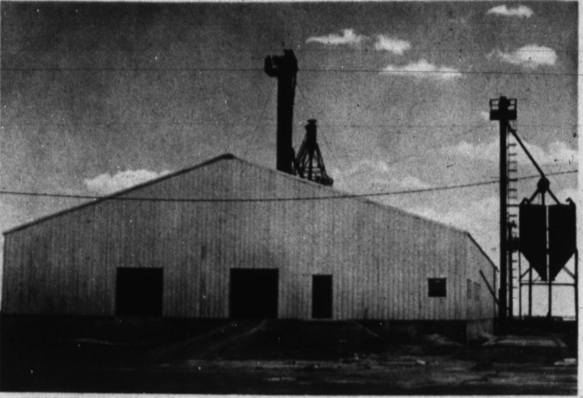
SWIFT AND CO. mineral block plant located by Progressive Road in Hereford is now being worked on its final stages before it is completed next month. (Hereford Brand Photo)
