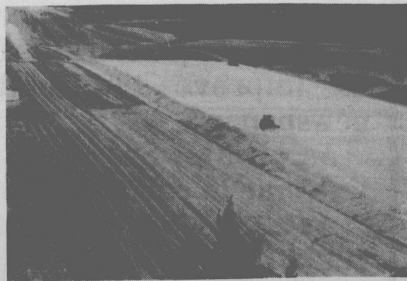
On Feb. 15, 1989, graders begin to level off a mound of earth.
