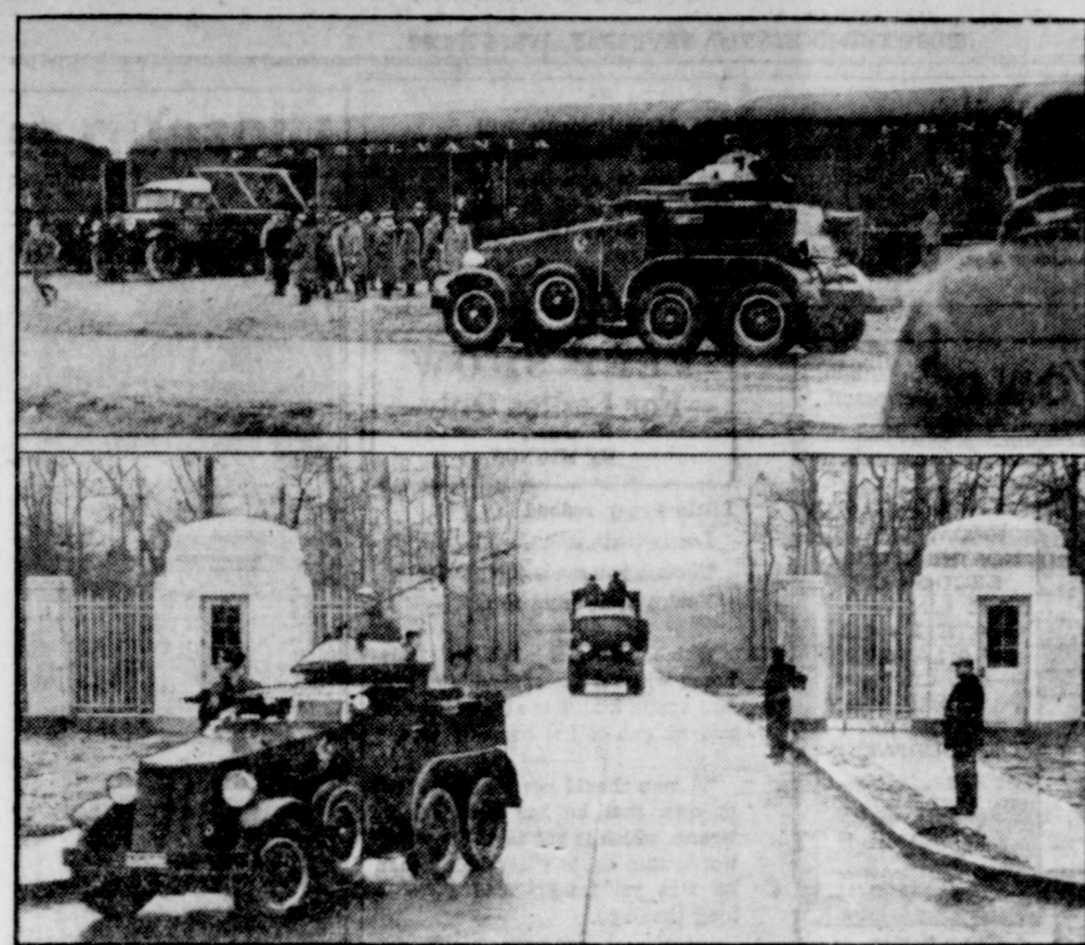
Utmost secrecy cloaked movements of the men, the trucks, and the train which transported half a billion dollars in gold bars from the Philadelphia mint to the new federal depository at Fort Knox, Ky. The upper picture shows the trainload of ingots arriving at Fort Knox. Below, an armored car with its deadly machine gun turret and its radio antennae overhead, moves before a bullion truck carrying a million dollars in gold from the train through the gates of the Fort Knox "pillbox."
