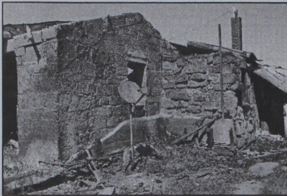
Photo at left: The original construction from the 1880s is on the right. The stone is rougher cut and part of the house is built into the bank. The 1890s addition is on the left.
