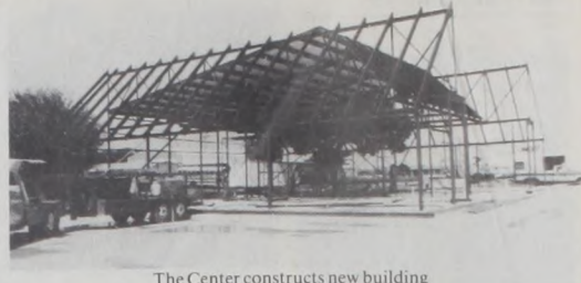
The Center constructs new building
