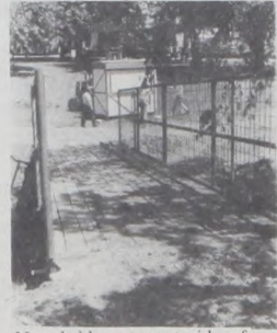
New bridge at west side of park
