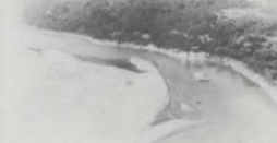
Proposed site for a Red River bridge
