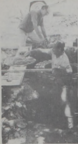
Manhole construction at Sacred Heart School.
