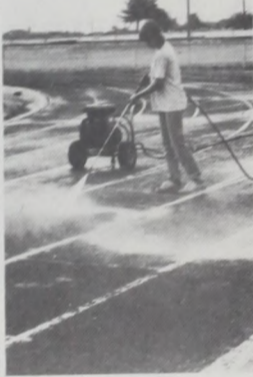
Resurfacing of MPS track.
