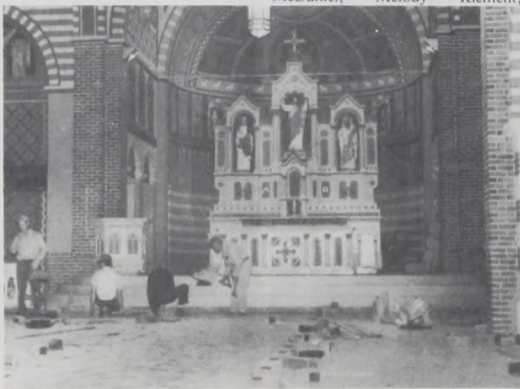
Restoration nears completion at St. Peter's Church of Lindsay.
