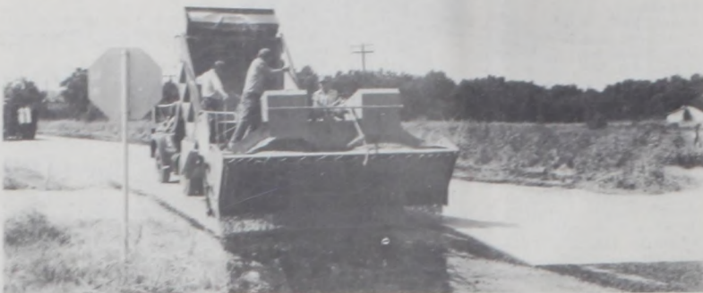
Eddy and Ash Streets receive paving.
