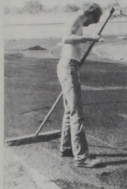
MIKE REITER smooths the first of four layers of rubberized material this week on the MPS track. Above, Shonna Reiter washed the track prior to the resurfacing work. The track will not be completed until next week.
