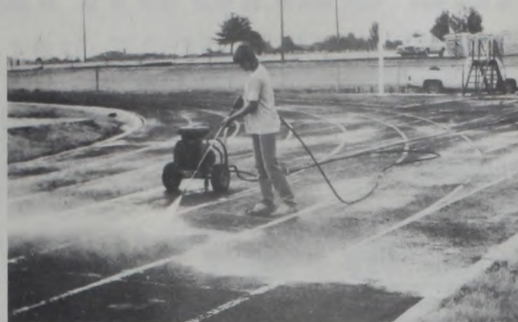
MIKE REITER smooths the first of four layers of rubberized material this week on the MPS track. Above, Shonna Reiter washed the track prior to the resurfacing work. The track will not be completed until next week.
