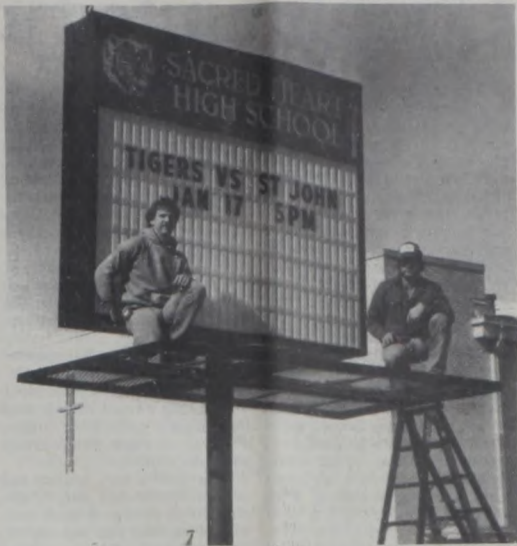
THIS HANDSOME ADDITION to Sacred Heart High School campus is the new lighted marquee near the gym. It was designed by Bert Hesse, shown at left, and constructed by Jesse Walterscheid, at right. The folding ladder is designed to hinge to the underside of the steel platform when not in use. Dave Fette Photo
