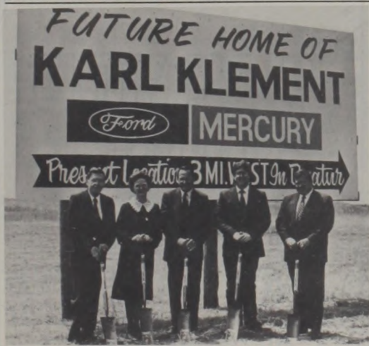
KLEMENT GROUNDBREAKING - Mr. and Mrs. Martin L. Klement, left, of Muenster were on hand Sept. 8 to help their son, Karl J. Klement, second from right, break ground for his new $1.2 million Ford-Mercury dealership facility in Decatur. Also helping shovel the dirt at the occasion were Dick Davis, right, Dallas District Manager for Ford Division and H.S. Feder, center, Dallas District Manager for Lincoln-Mercury Division.
