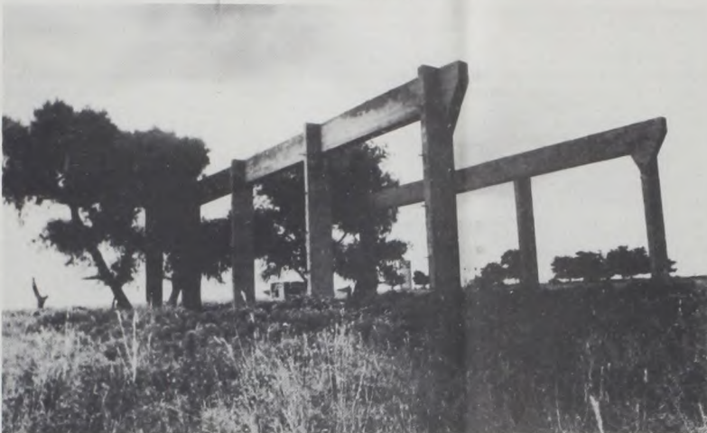
ALL THAT REMAINS of a large warehouse, where supplies were unloaded from a train before re-distribution at Camp Howze, are these huge concrete support beams. Janie Hartman Photo
