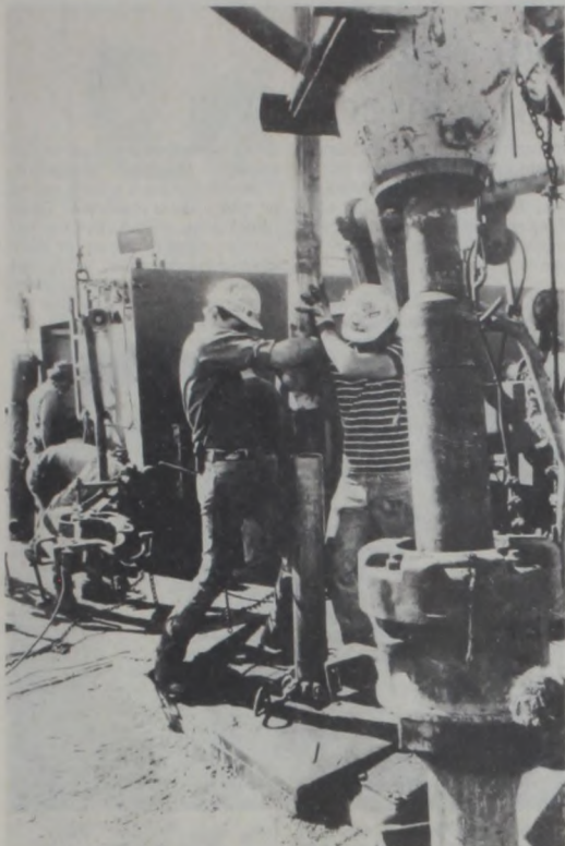
LOCAL DRILLERS stayed busy for the past two months, but exploration in the immediate area has slackened, because of the prospects of drilling a profitable well. Felderhoff Production started drilling Wednesday on the Trachta Lease, east of Muenster. Bill Harris and Bill Haverkamp, crew members, connect joints on the rig. Janie Hartman Photo
