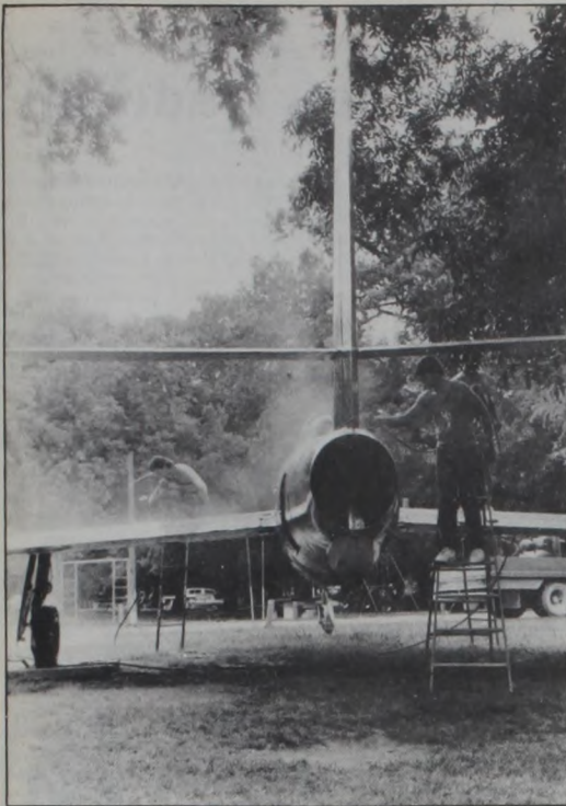
THE LAST FEW MONTHS , the Muenster Jaycees have been repairing the F-84-F Thunderstreak jet plane in the Muenster City Park. With the vandal-induced holes patched, the plane sanded and cleaned, the obsolete Korean War plane was ready to paint. David Muller and Darren Voth are shown applying the gray paint. They were helped by Bret Walterscheid and Ron Trubenbach. The Jaycees plan to return the original decals to the airplane for a more authentic appearance. The Jaycees installed the plane in 1971.
