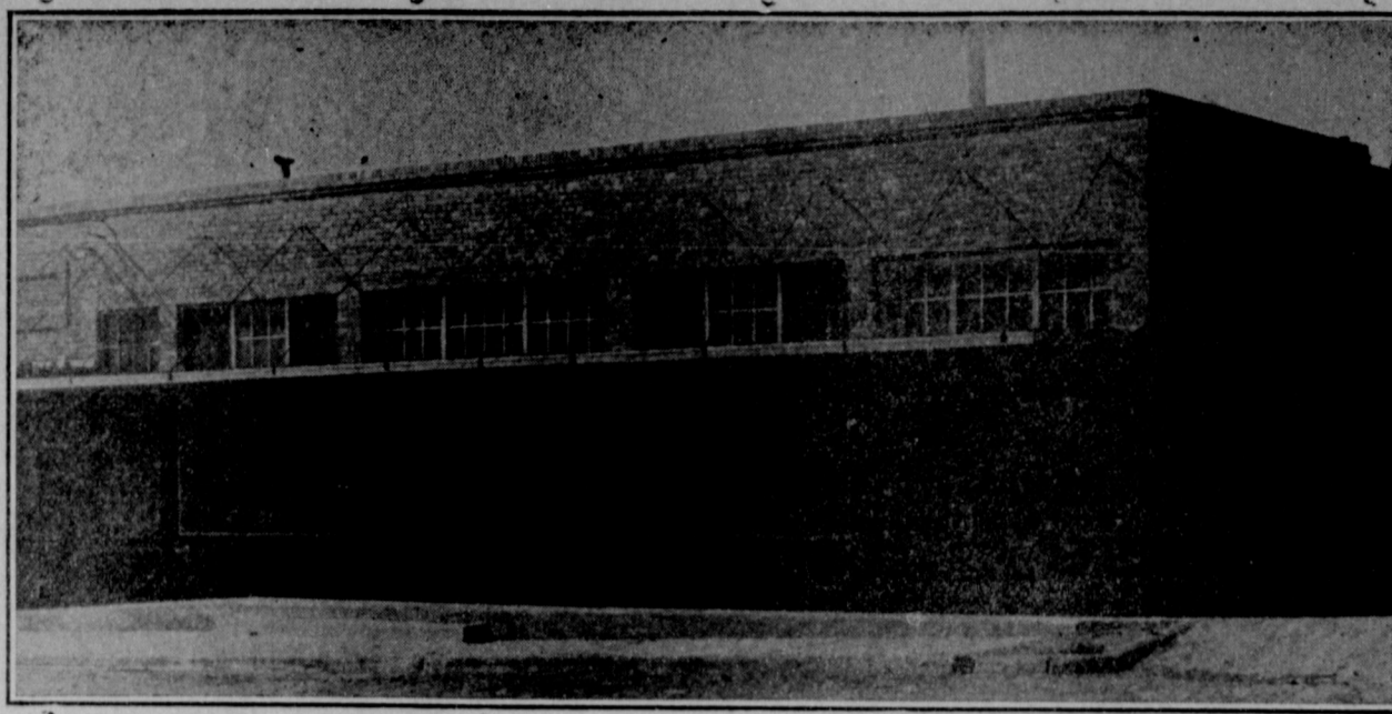
FMA Store Building Completed October, 1939
