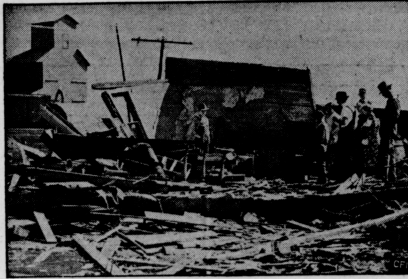
More than 125 people were injured and at least 41 were killed. The tornado, or series of them, started in Texas and swept through Oklahoma and Arkansas during the week-end. The loss of property damage is inestimable. This picture shows the damage in Capron, Oklahoma, where seven persons were killed and 33 injured. The damage to property was estimated at $200,000.
