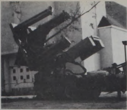
The accompanying photo shows work progressing as two Red Oak trees are being planted in front of Sacred Heart Church. David Bayer prepared the holes with his "Diggin Dutchman" equipment, and did the planting. The Catholic Life Insurance Union, Branch No. 18 paid for the work and the trees.
